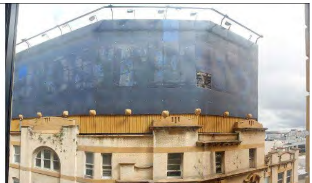
Existing situation – view from adjoining hotel
