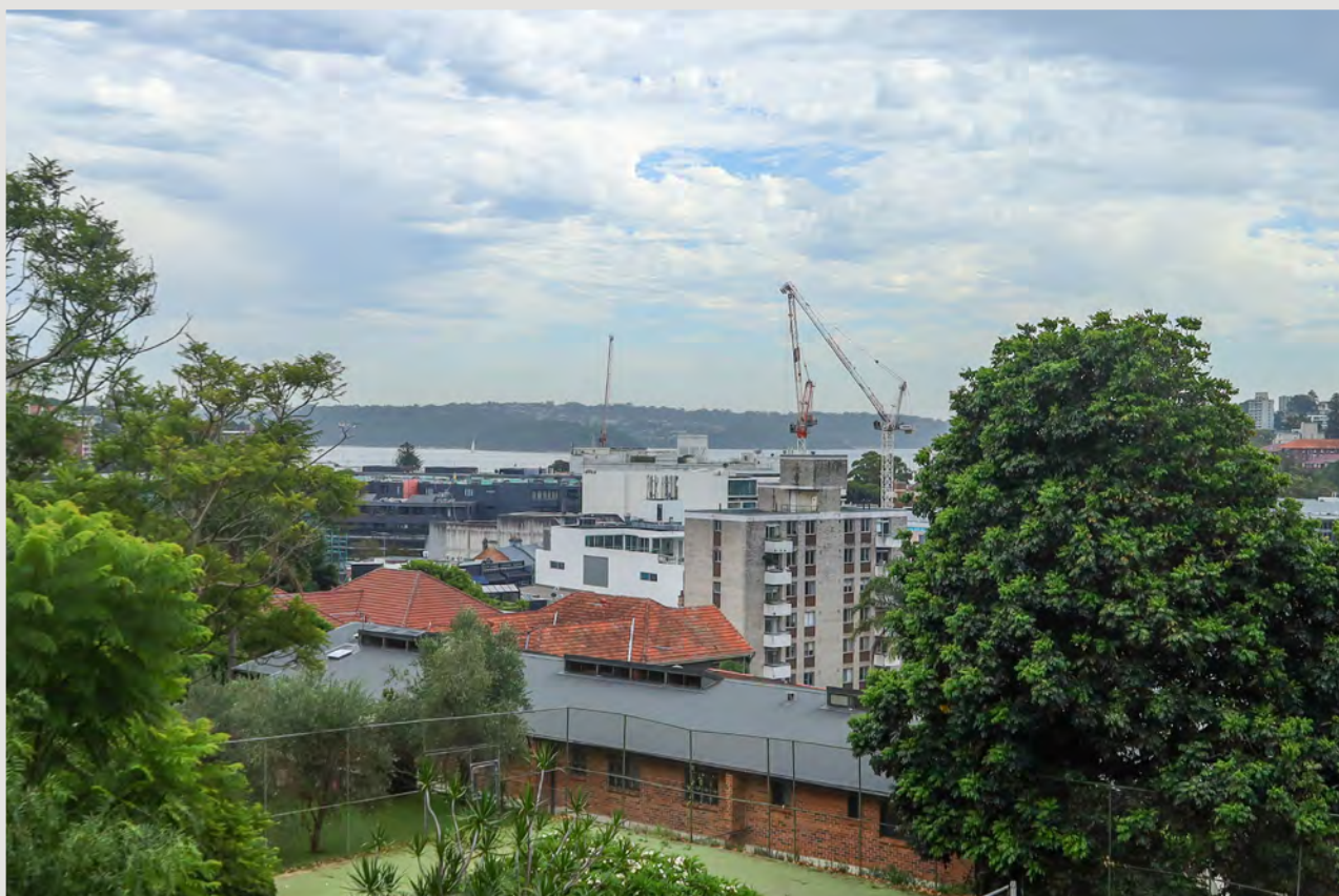
Existing site photo - No.10, Pine Hill Avenue.
