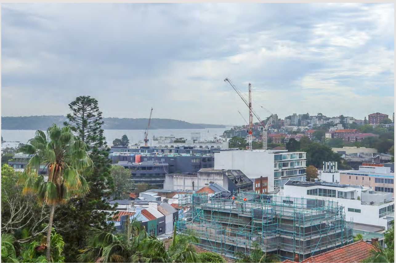
Existing site photo - Unit 603, 349 New South Head Road
